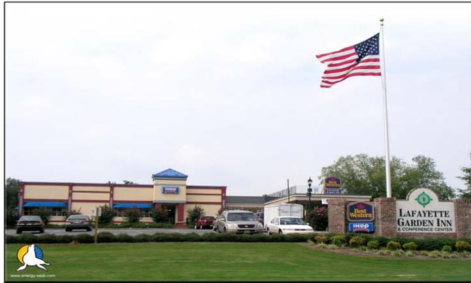
The Energy Seal Coatings EPDM roof coating system was specified and installed on this project.
