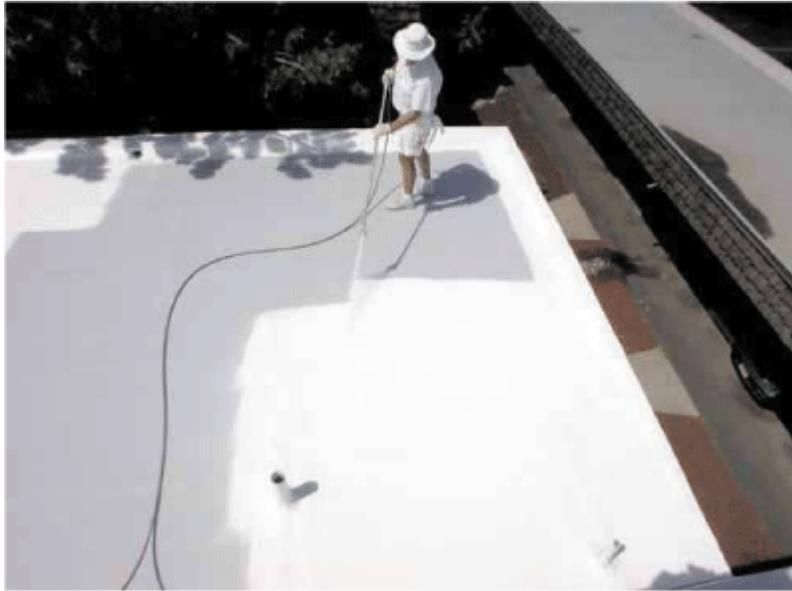
White coatings - The white coating is sprayed over a base coat on top of an old built-up roof Source: Interface, February 2007
