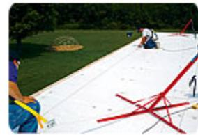
PREFAB Custom prefabricated single-ply roofing systems are precisely measured in advance to fit each roofing job. This virtually eliminates membrane material waste and several trips to the local landfill. It also reduces labor requirements and installation times, and minimizes the risk of human error by performing up to 85 percent of the seaming in the factory under controlled conditions. (Photo courtesy of Duro-Last Roofing Inc.)
