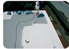
APARTMENT ROOF Photo courtesy of United Coatings, an RCMA member.
