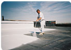
SPRAY APPLICATION Photo courtesy of Gardner-Gibson Inc., an RCMA member.
