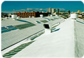
COMMERCIAL ROOF Photo courtesy of United Coatings, an RCMA member.
