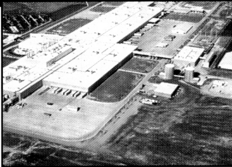
Light colors are an effective means of reducing the peak demand for cool energy in buildings.
