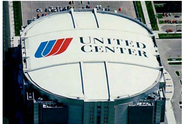
100 m 2 (~1000 ft 2 ) of a white roof, replacing a dark roof, offsets the emission of 10 tonnes of CO 2
