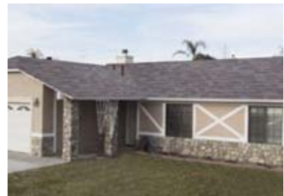
Before: Hot roof, with gray asphalt
