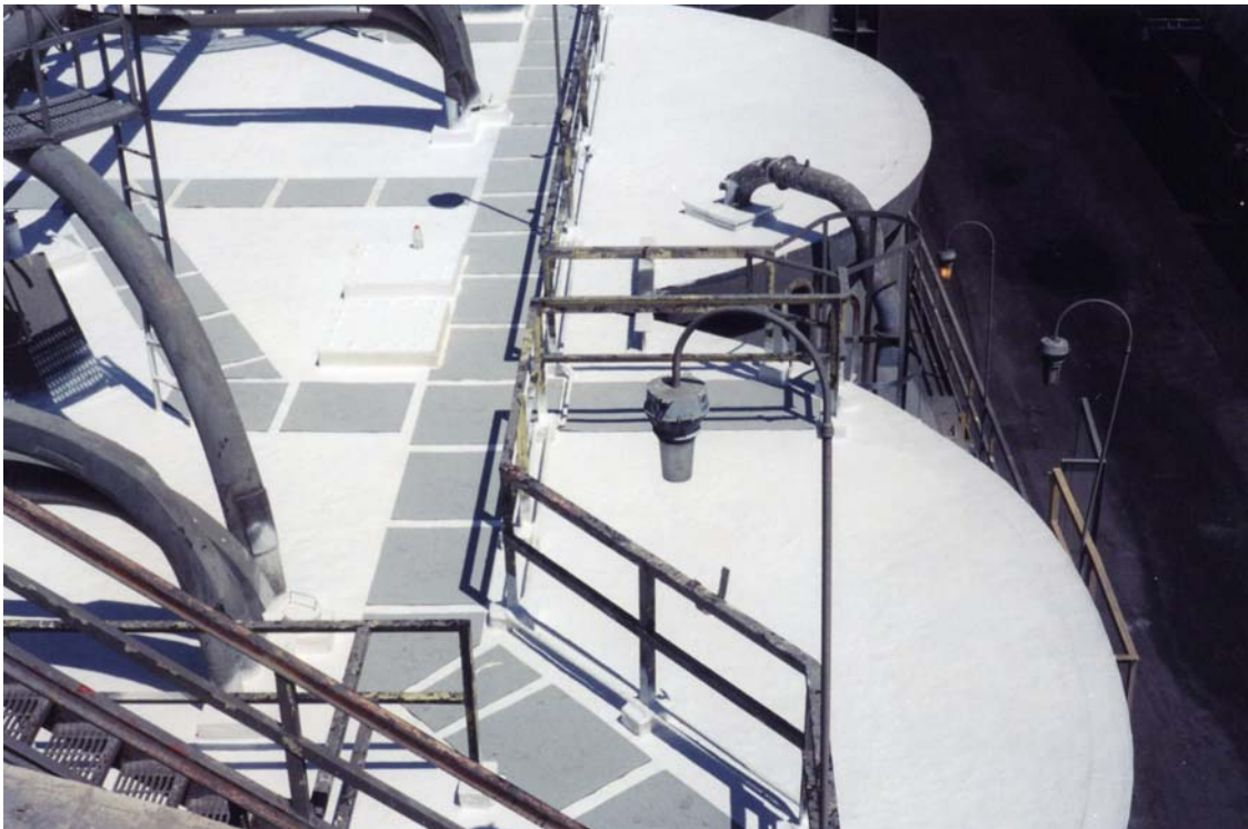
The roof with walking deck installed
