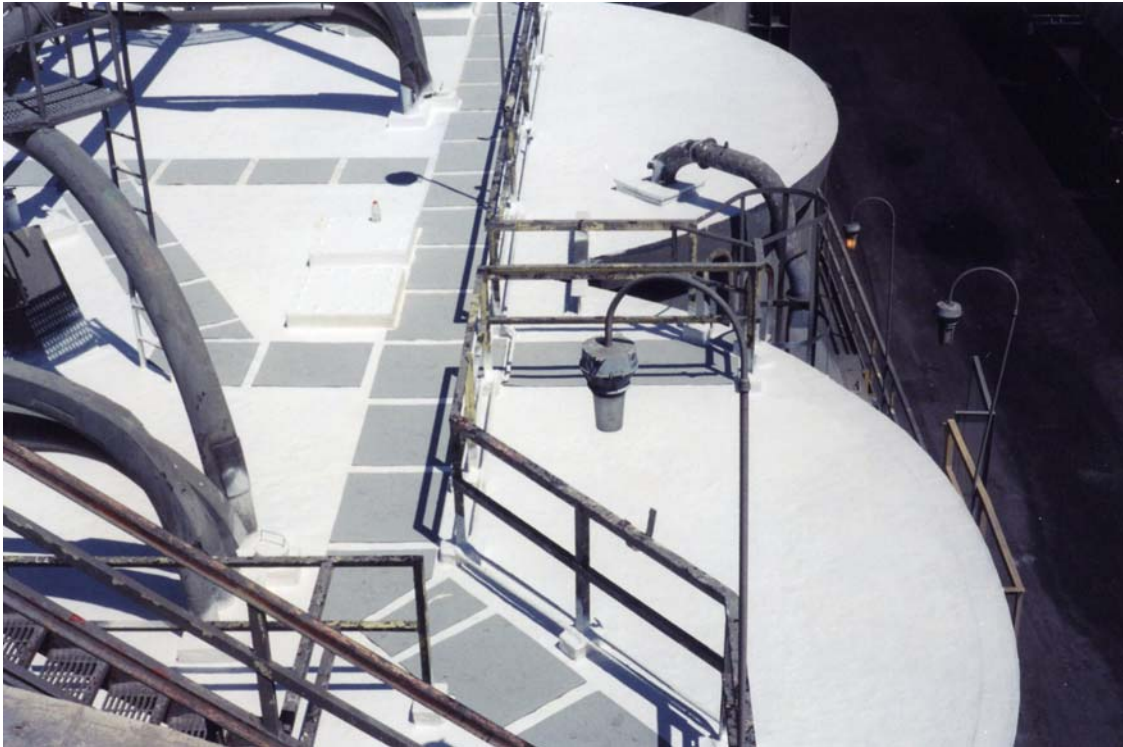
The roof with walking deck installed
