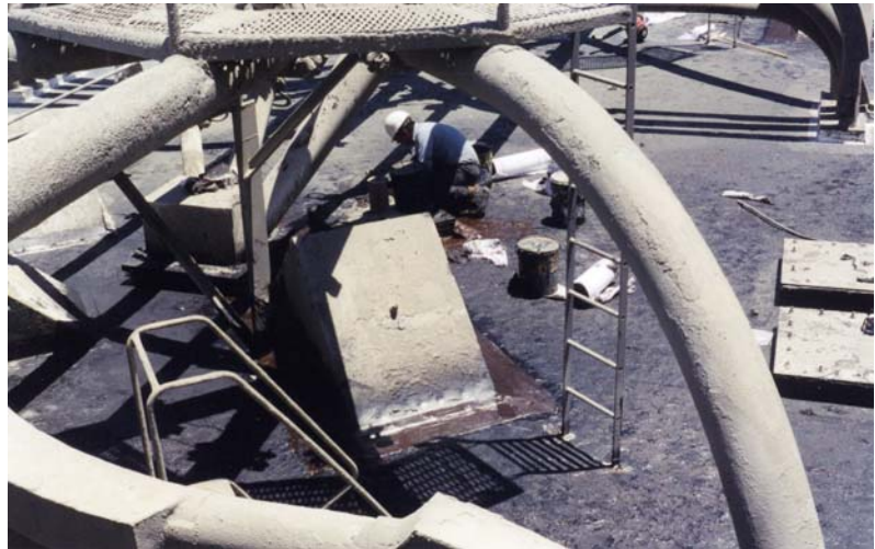
Equipment and flashings are prepared on the primed roof deck.
