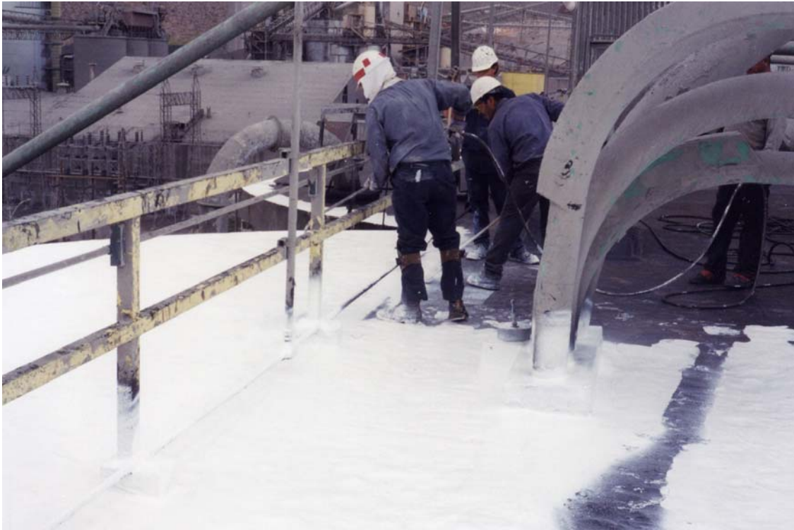
Spraying the first layer of Energy Seal's Acu-Shield onto the roof deck
