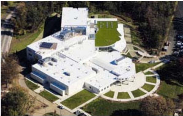
The R&D agreement's objective is the development of new technologies that would enable cool-roof manufacturers to meet a standard of 75% solar reflectance after five years.
