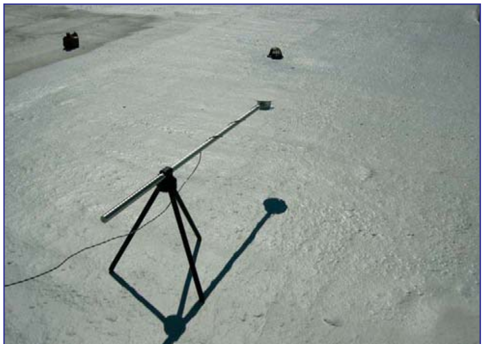
Figure 1 – Albedometer measuring foam roof reflectivity.
