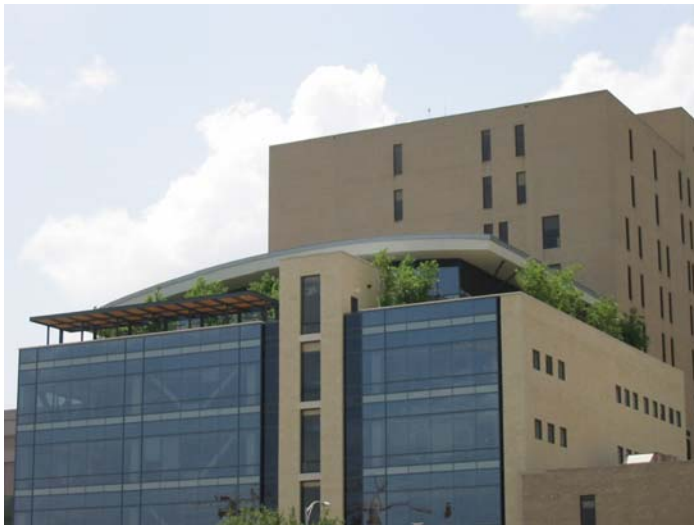
The South Texas Law School garden roof provides greenspace for employees and students as well as cooling this part of the roof structure.
