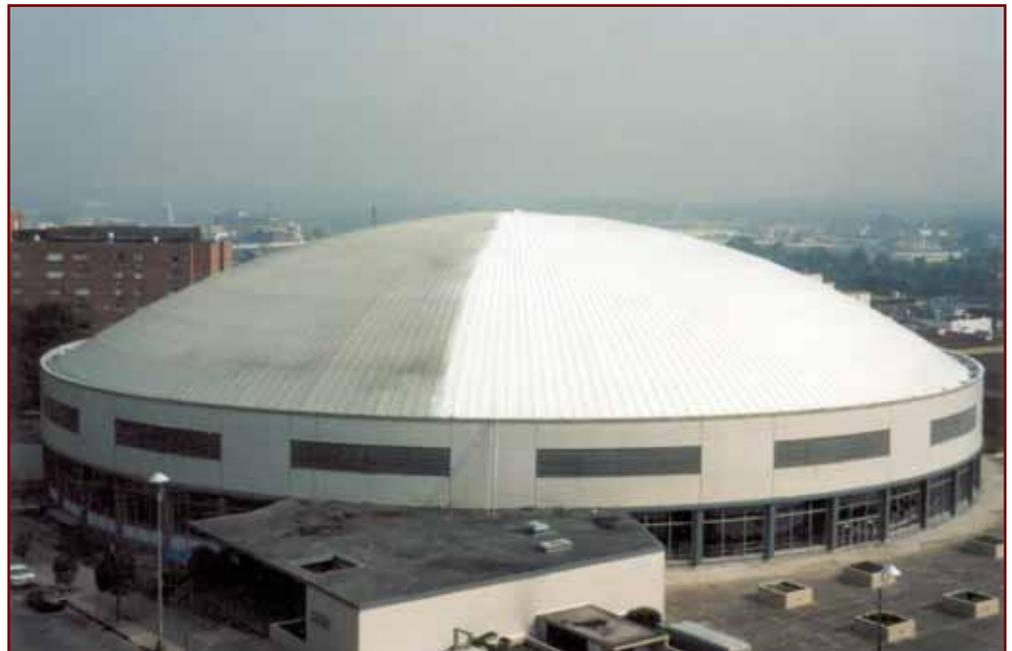
*This metal roof at Eastern Tennessee State University is partially covered with a white coating. The coated half of the dome contrasts sharply with the uncoated half mid-way through the application process.*
