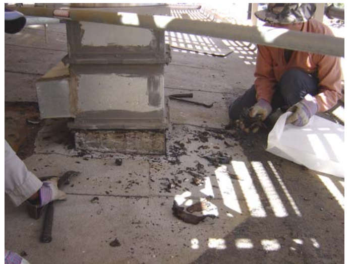
All vents and pipes are scraped down and prepared for the Energy Seal's Acu-Caulk: Brush Grade.
