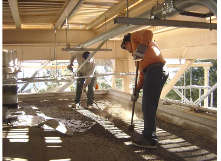
Rock is spudded off and removed.
