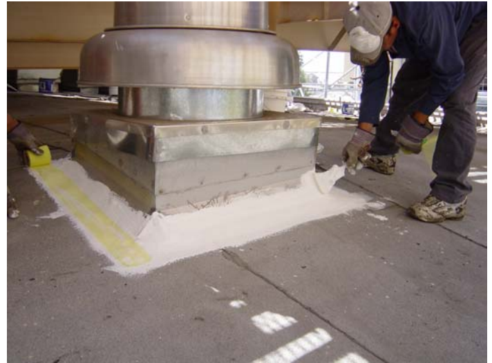
Elastomeric cement is reinforced with fiberglass around all vents.
