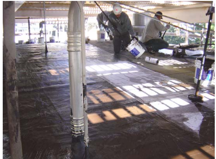
Installing polyester and rubberized emulsion.
