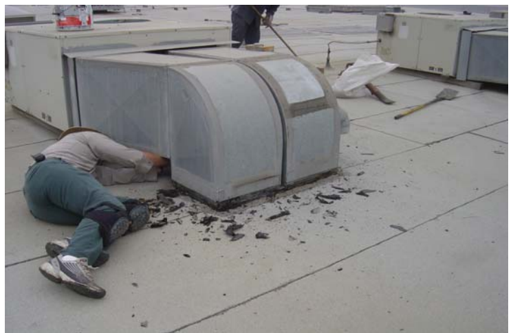
All penetrations are scraped down.
