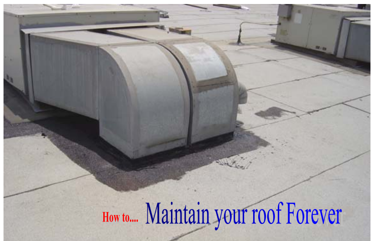
All penetrations are primed to create a solid long lasting bond to the new maintenance roof.
