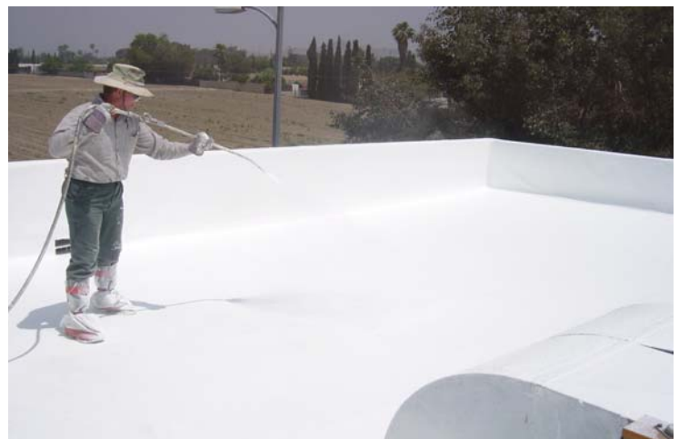
2 layers of Acu-Shield white coating are sprayed onto the roof. This will reduce temperatures and save money.
