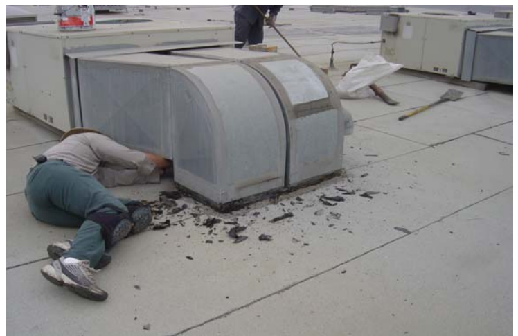
All penetrations are scraped down.
