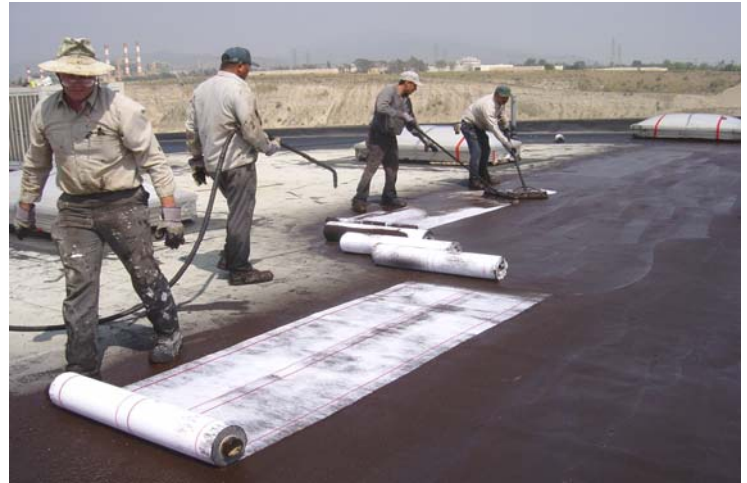
2 layers of extra tough Acu-Fabric are bonded to the existing roof.
