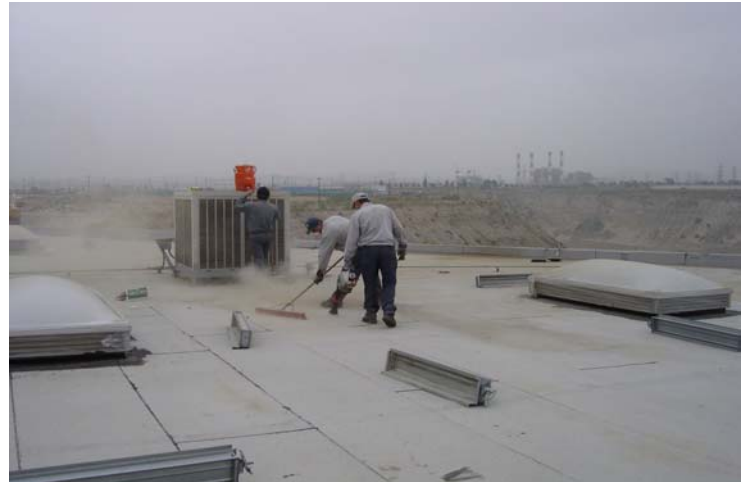
Cleaning the roof for the new polyester and emulsion roof system.
