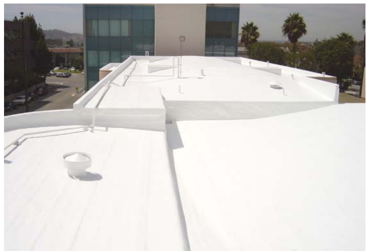
The finished roof.
