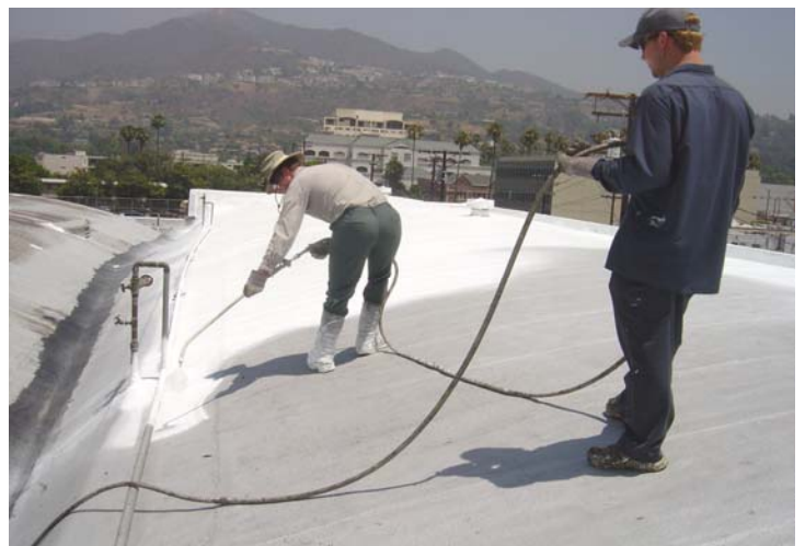
The first of three layers of Energy Seal Acu-Shield white acrylic coating is applied.
