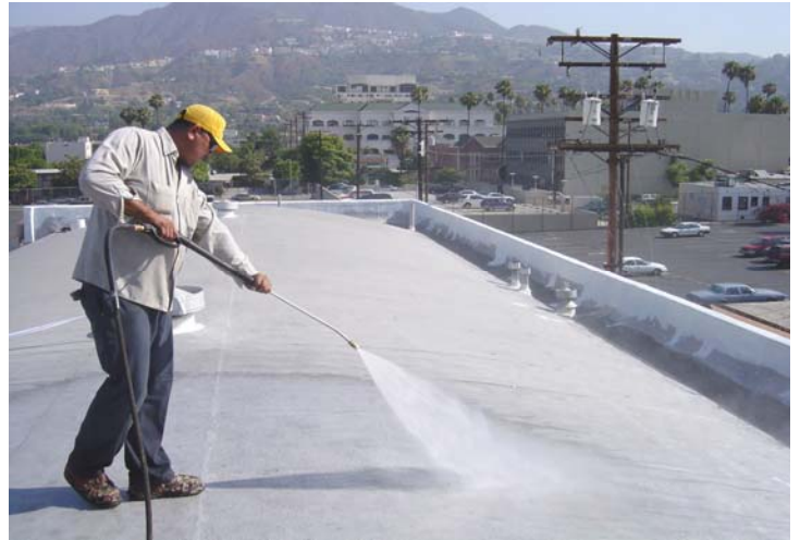
Before coating, the roof was power washed.
