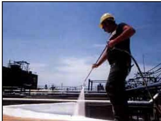
Elastomeric roof mastics based on RHOPLEX EC acrylic prolong the life of polyurethane foam by protecting it from ultraviolet degradation.
