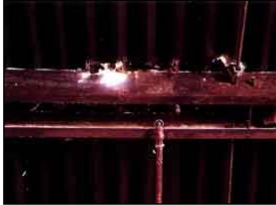
Constant expanding and contracting of the metal roof due to temperature changes led to splits in the panel seams. This photograph was taken from inside of the building looking up.
