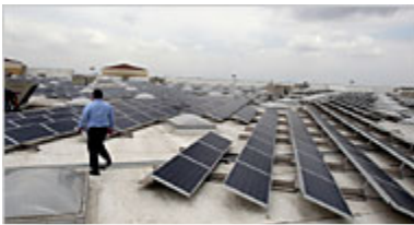
J. Emilio Flores for The New York Times A Wal-Mart store in Chino, Calif. has both a cool roof and solar panels to cut its energy use.
